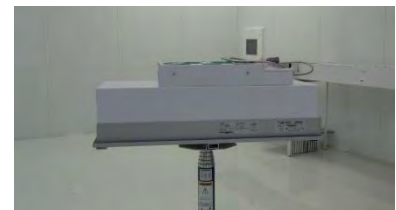
Figure 2. FFU shown on top of lifting hoist.
