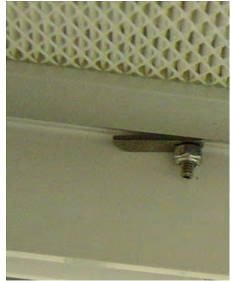
Figure 1. Non-walkable bottom load filter clip shown rotated out of the way for filter installation. Rotate out perpendicular to grid and tighten nut.
