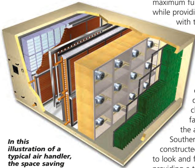
*In this illustration of a typical air handler, the space saving advantage of FANWALL TECHNOLOGY over a typical single fan is apparent. Also, because of the multiple-fan design, the downstream airflow is smooth and uniform.*
