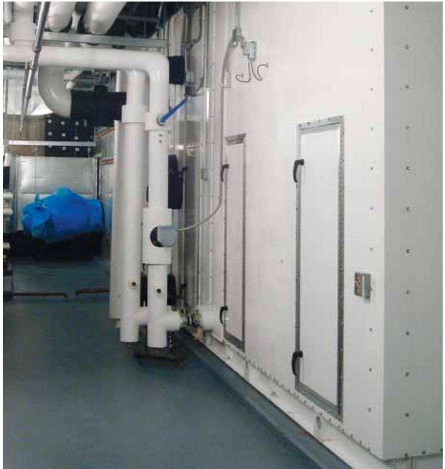
*Even though they were brought into the mechanical room in piece parts, the installed HUNTAIR® air handlers looked as if they had been factory-assembled.*
