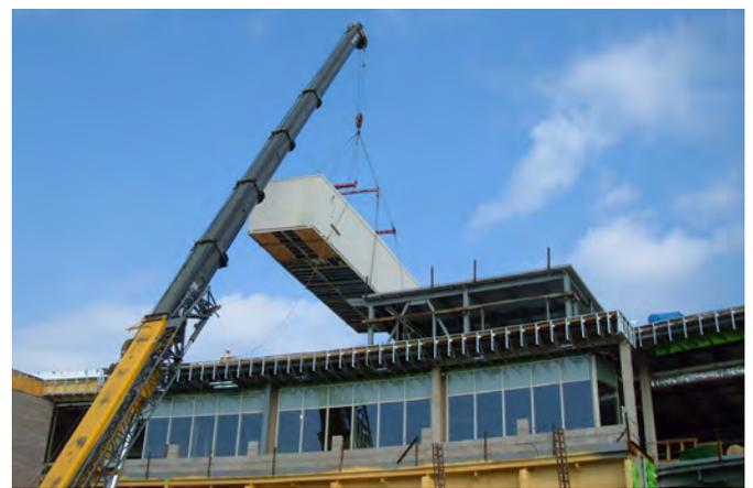
**The rooftop system on the new facility provides 151 tons of cooling and 8,000 MBH of heating. It also provides 200 MBH of domestic water heating for both facilities with a 500 gallon storage tank.**
