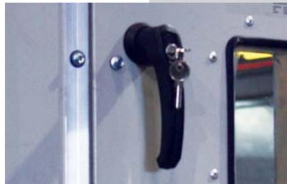
Handles are a **thermal bridge issue**. Hands can get scraped with door handle. External handle mounted on unit casing.
