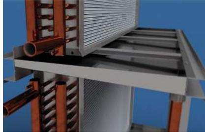
Auxiliary drain pan has potential for water overflow.
