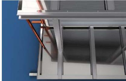
Cascading auxiliary drain connections can cause the lower auxiliary drain pan to overflow.
