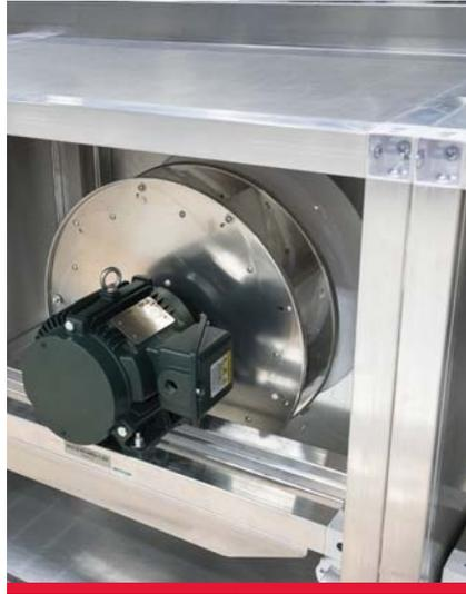
**Only option is to ramp up and down the entire fan array.** This is inefficient as it runs the motors in the bottom of their efficiency curve to achieve lower CFM output. This becomes costly both in kWh and maintenance.
