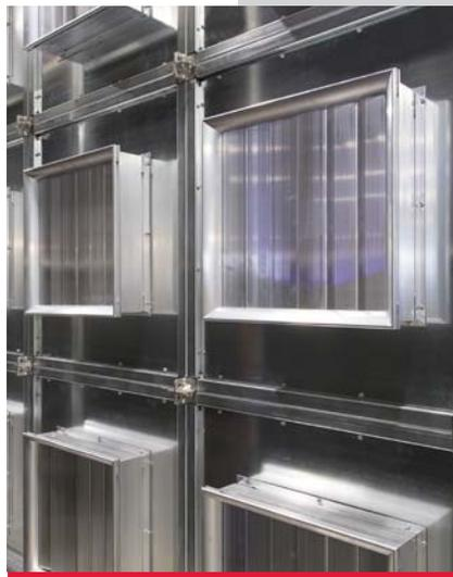
**Open inlet with no prevention for recirculation.** If a fan goes down, the cell with the inoperable fan will see significant recirculation of air decreasing the efficiency of the air handler while also creating turbulence in the airflow.
