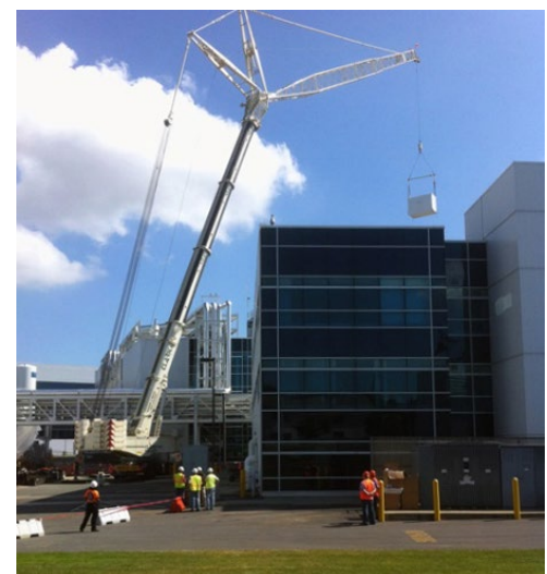
Ventrol sectional unit construction makes installation possible in hard-to-reach places.
